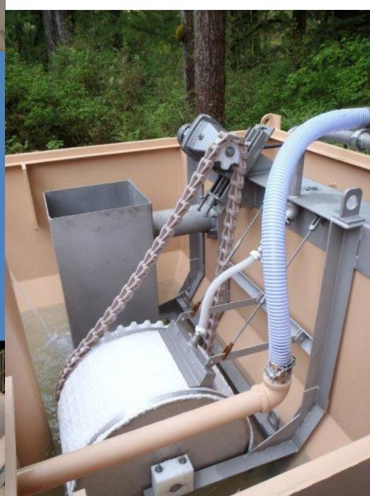
The **BioDRUM™** filter will produce reuse quality effluent,
