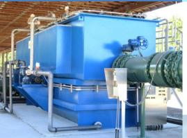
Wastewater Technologies continues to expand its liquid/solid separation capabilities by adding a user-friendly, small footprint, low backwash, high performance tertiary filter for both small and large flow applications. The **BioDISC™** Cloth Media Filter removes suspended solids as small as 10 microns and can be configured for flows as low as 100,000 GPD to over 6 MGD.
